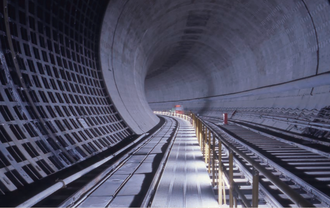
Kanda River / Kandagawa Ring Road No.7 (Kannana-Dori) Flood Control Reservoir
